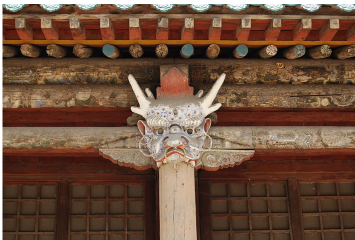
Obr. 2.2-3: Horné časti stĺpov ( dougong ), jaskyne Yungang , provincia Shanxi, prevzaté od Marcin Bialek; Top of the Column in the Building Protecting the Caves of Yungang Grottoes, Datong, China ; 23 July 2010; Web; 15 Feb. 2013.
